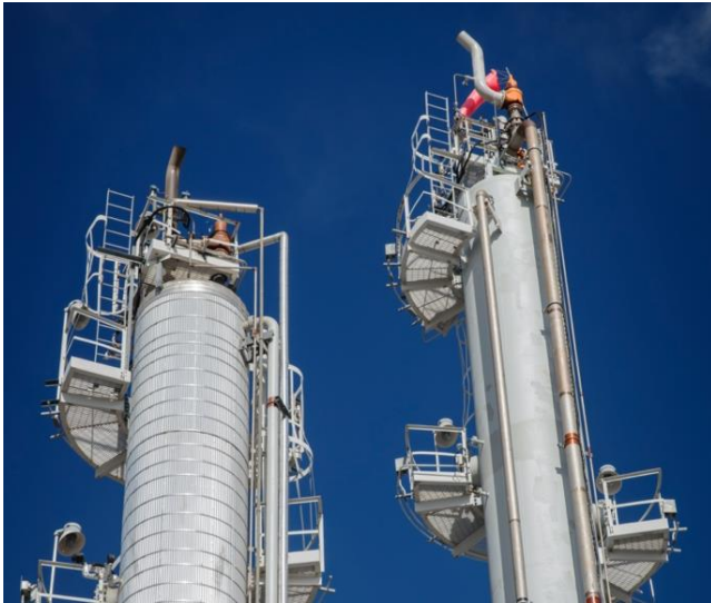
Example of a chemical plant distillation tower. Certain process vents associated with distillation and other processes that manage hazardous waste may be subject to Subpart AA.
