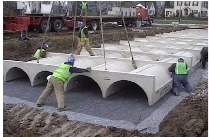
Installation of a subsurface stormwater storage and infiltration gallery.
