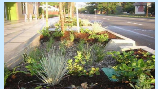
When this bioretention planter box is full of stormwater, the extra water "backs up" into the street to drain into a storm inlet.
