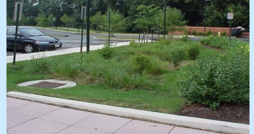
A storm inlet is used in this bioretention area to drain overflowing stormwater.
