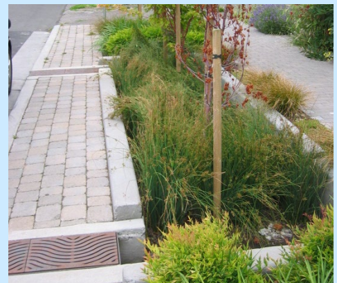
This roadside bioretention collects and treats roadway stormwater.
