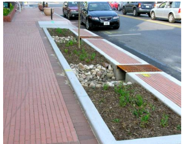
This roadside bioretention captures stormwater from the road. The paved shoulder and metal grates provide roadside parking access.
