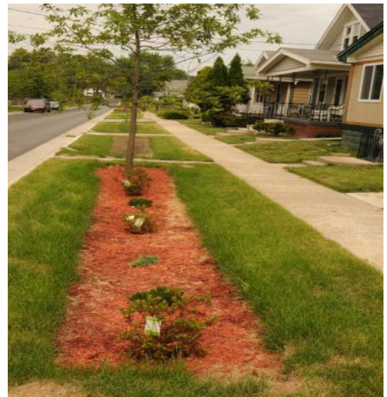
Roadway and sidewalk stormwater drains to this roadside bioretention system on Maywood Avenue in Toledo, Ohio.
