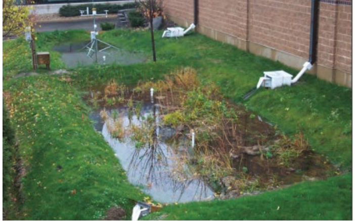
Roof stormwater drains to these monitored rain gardens in Madison, Wisconsin.
