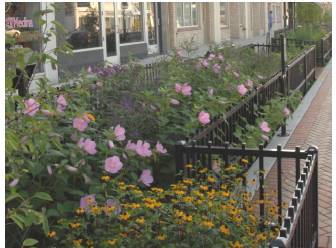
Bioretention planter boxes in Lansing help treat stormwater from roads and sidewalk.
