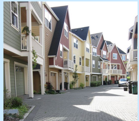
Stormwater drains through this permeable paver drive to a stone storage layer.
