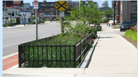
This bioretention planter box was designed into a pedestrian corridor.
