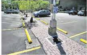
SLOWING RUNOFF Porous bricks in a parking lot help prevent sewers from overflowing.
