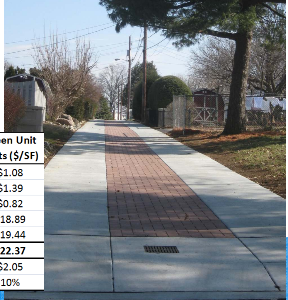
Green alley retrofit (permeable pavers with infiltration trench)
