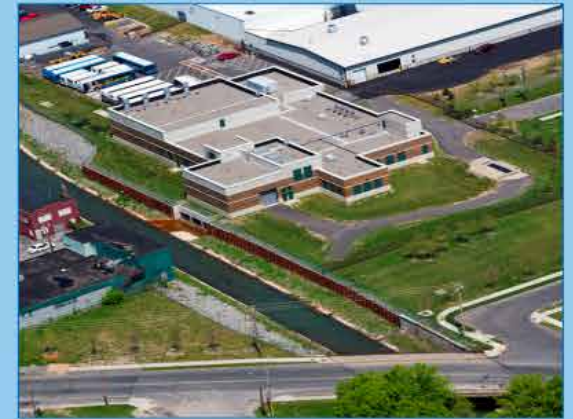
Midland Avenue Sewage Treatment Plant
