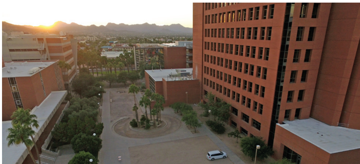
Figure 16 - Aerial view of existing site conditions
