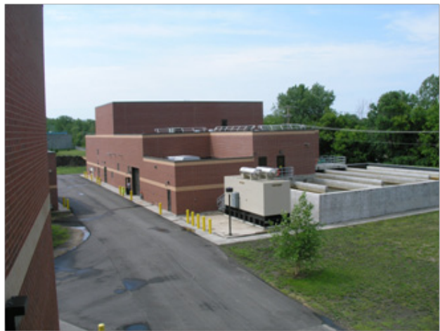
Figure 5-21 Mankato Water Reclamation Facility
