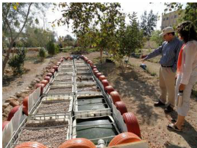
Figure 2 Graywater reuse system
