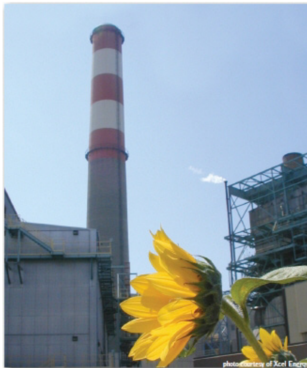
Figure 1 Cherokee Station (Photo credit: Xcel Energy)
