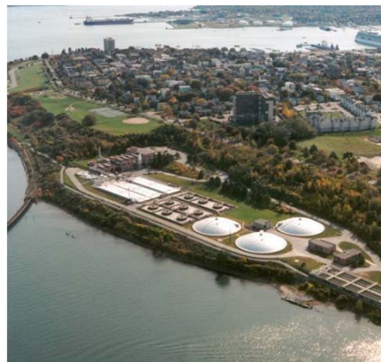
Photo Courtesy of Portland Water District
