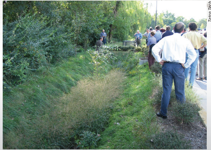
Visitors learn about a roadside rain garden from experts at the University of Maryland, College Park
