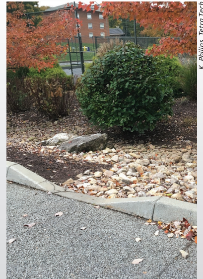
Local zoning code allows for curb cuts, Harrisonburg, Virginia
