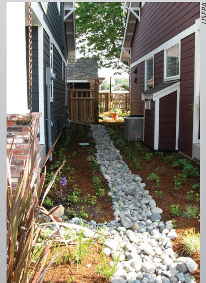
Zoning code allows for LID practices and limited setback between homes, Seattle, Washington
