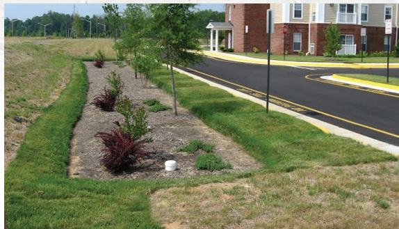
Stormwater infiltration trench, Stafford County, Virginia
