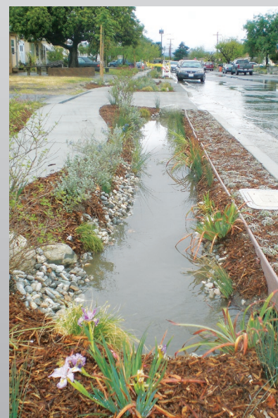
Sidewalk retention area, Los Angeles, Calif.
