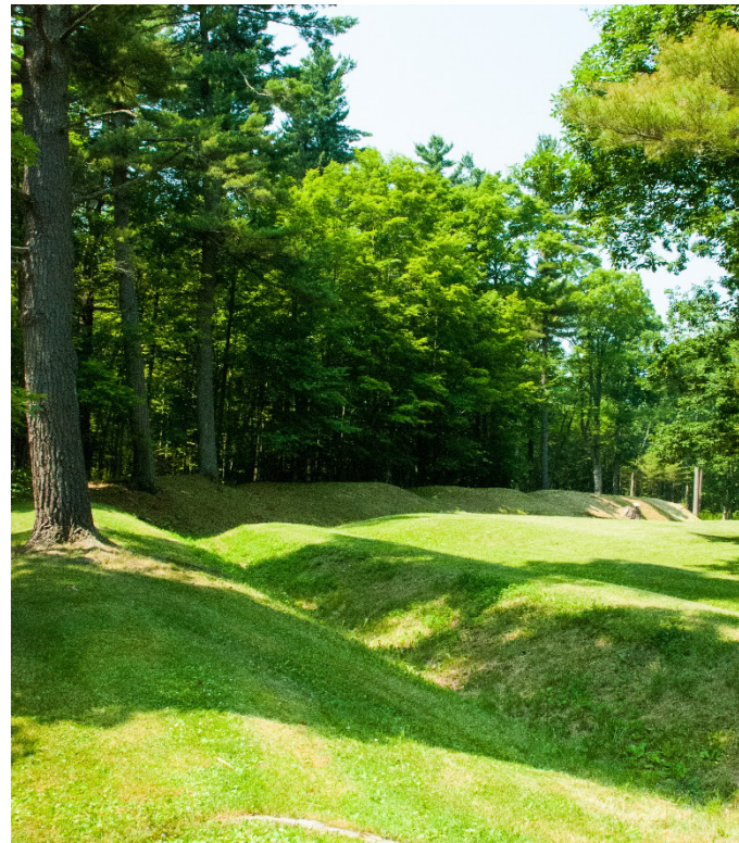
A grassed swale directs the flow of stormwater and allows stormwater to infiltrate.
