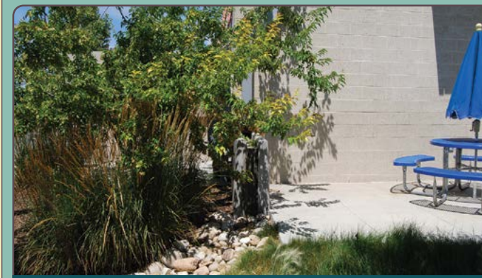
This system to divert rooftop runoff to a rain garden creates an interesting feature at this public library in Boise, ID.
