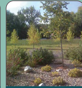
This rain garden in Denver treats runoff from a small area of pavement at an office facility. Note the incorporation of a tree in the landscaping
