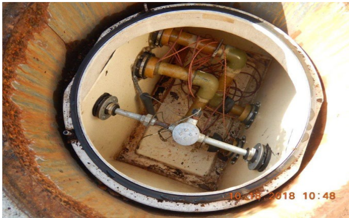
Figure 6.5. Cable in sump. Courtesy of Tennessee Department of Environment and Conservation.
