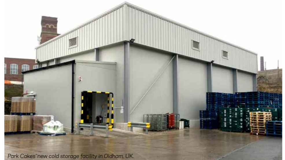
Park Cakes' new cold storage facility in Oldham, UK.
