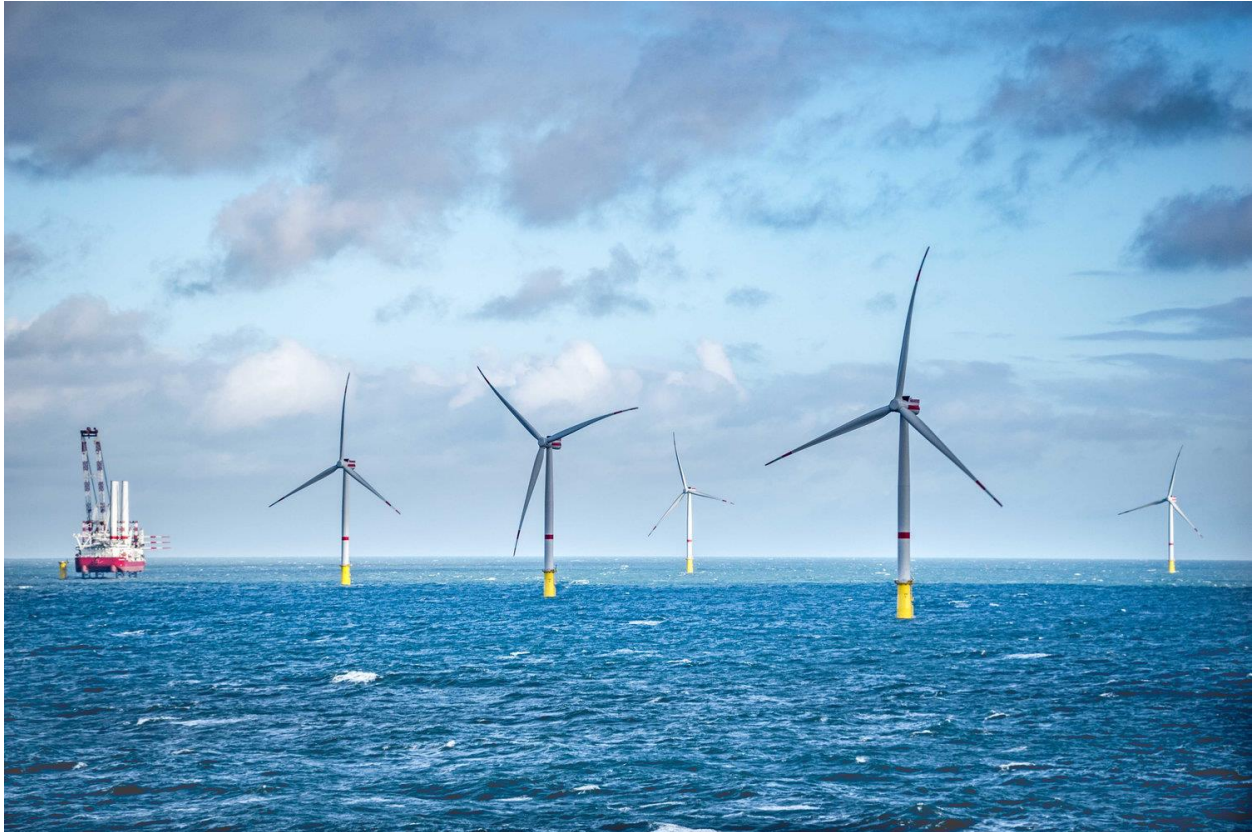
Figure 5. Example of Offshore Wind Turbine Generators with Monopile Foundations (for informational purposes only)
