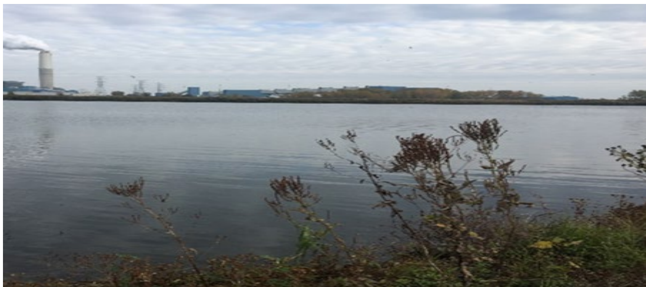
Photo 3: Typical Coal Ash Surface Impoundment Used for Storage and Disposal of Coal Ash: Surface impoundments can be quite large, with some units reaching upwards of 500 acres. Credit: U.S.. EPA
