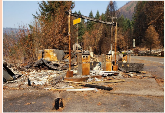
The Rivers Run facility after it was destroyed by the Lionshead fire
