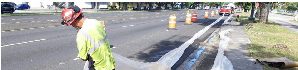
Crews servicing the sewer line along Route 1, Marine Corps Drive
