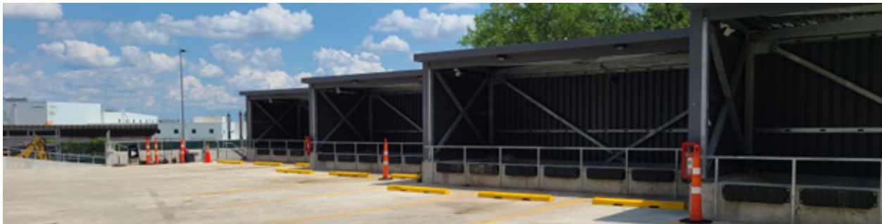
New elevated and covered disposal area at Trash Transfer Station
