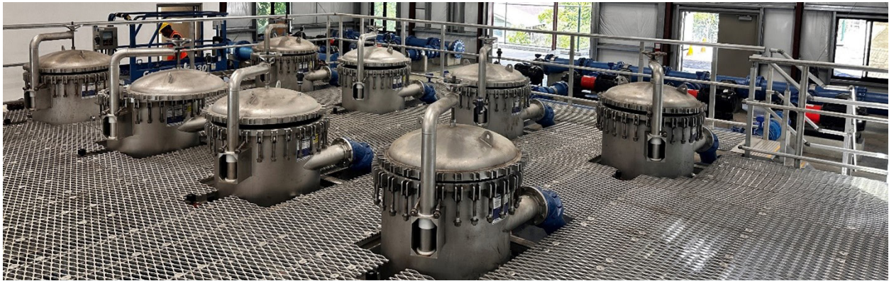
New ASPA sewage system and storage building.
