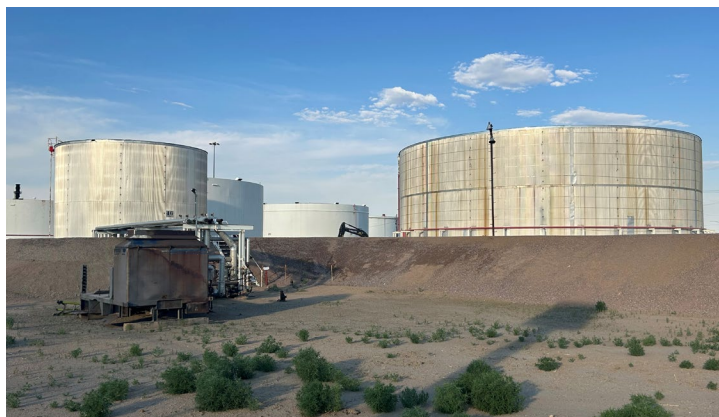
Suncor's Commerce City Refinery with a raised dirt secondary containment wall around the storage tank area.
