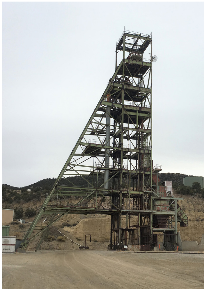
Head frame at Mt. Taylor before demolition
