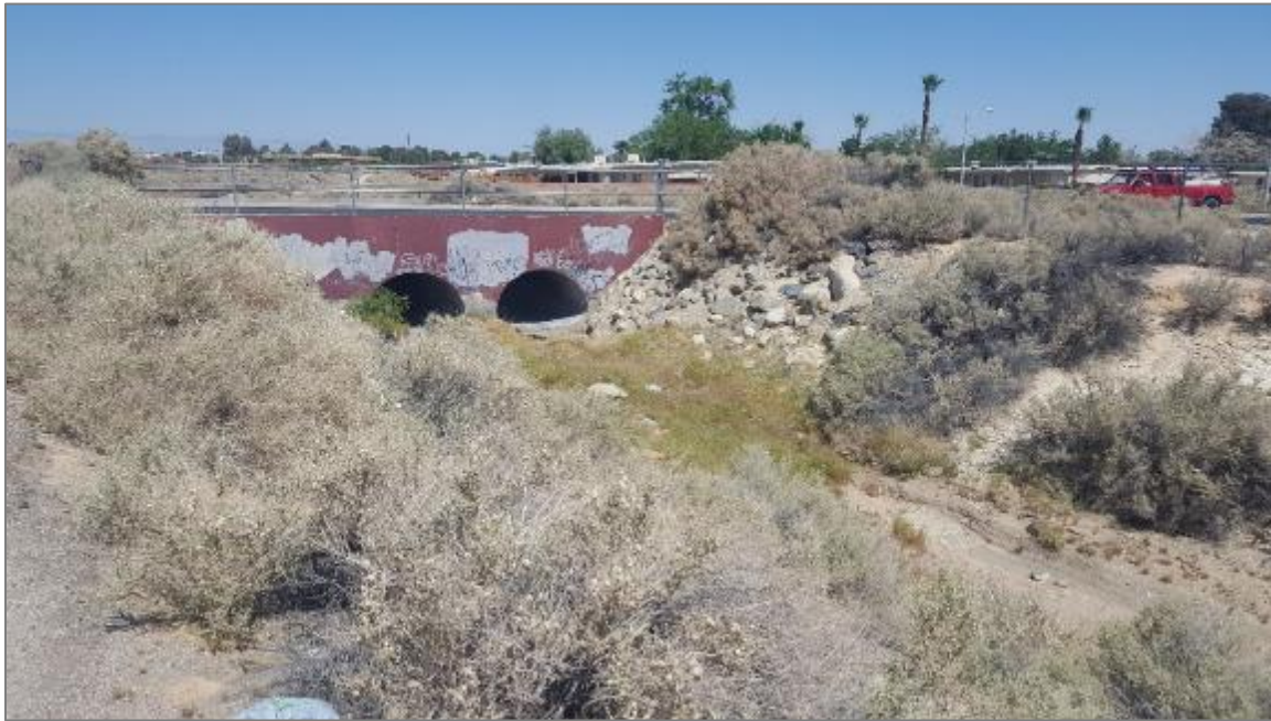
Figure 11. Local conditions that support growth of hydrophytes. In Ridgecrest, California, a culvert at an ephemeral stream crossing disrupts the movement of water, sustaining the growth of hydrophytes in the immediate vicinity. Photo credit: Cara Clark.
