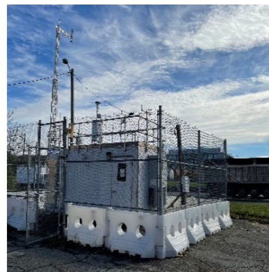
DC DOEE Anacostia site
