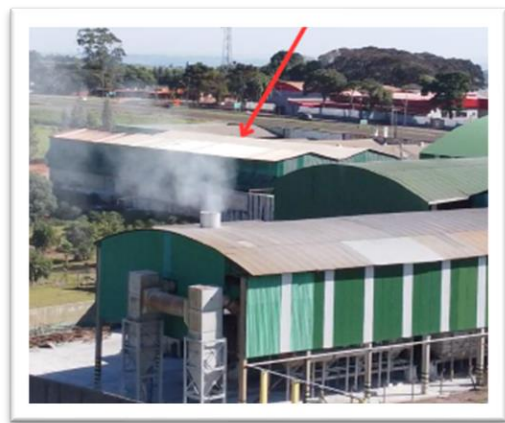
Licensed and unlicensed companies carrying out contamination
